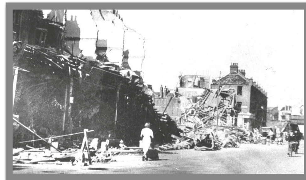
▲ Bomb damage along Beckenham Road August 1944
