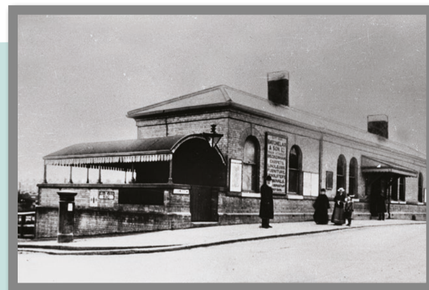
▲ Clock House Station 1890s
